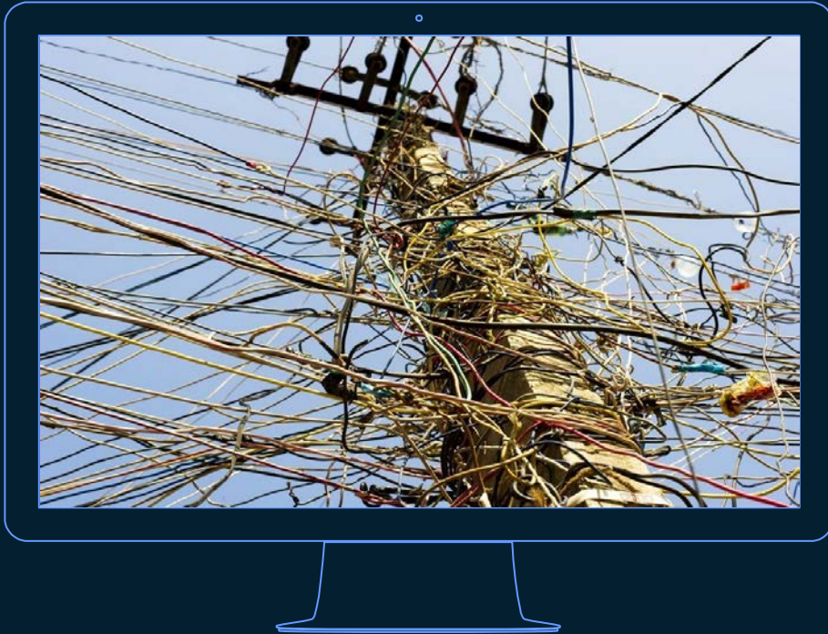
Power lines in India.
